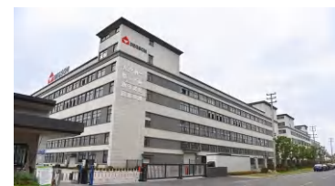
High-tech Zone Factory
